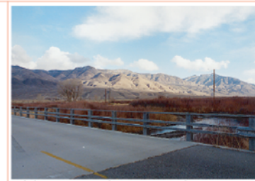
Highway 6 crossing Owens River.
