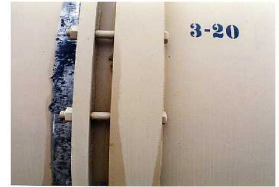
Splice-junction on pipe.
