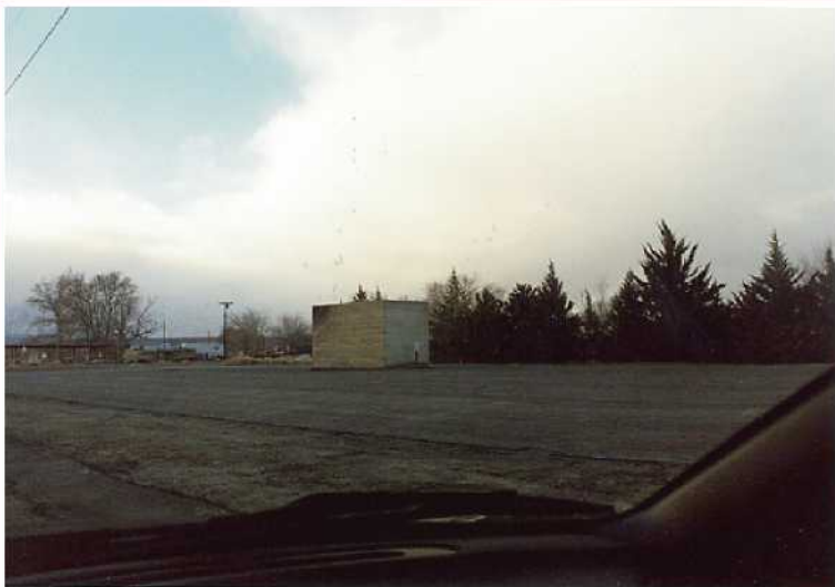
Concrete bunker, Laws.
