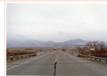
Highway 168 crossing Owens River.
