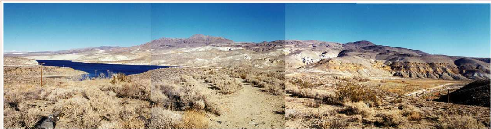
Haiwee Reservoir drains through a pipe rather than the outmoded stream bed.
