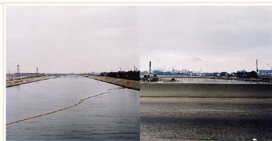
LA River from Ocean Boulevard, Long Beach. The drag line prevents victims from being swept out to sea.
