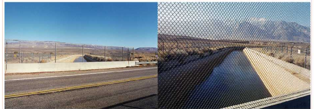
Final stretch of the open concrete-lined canal north of Haiwee.
