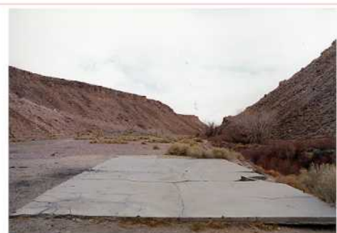
Slab at bottom of Pleasant Valley dam.
