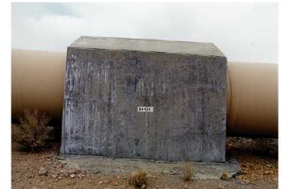
Splice-junction on pipe.
