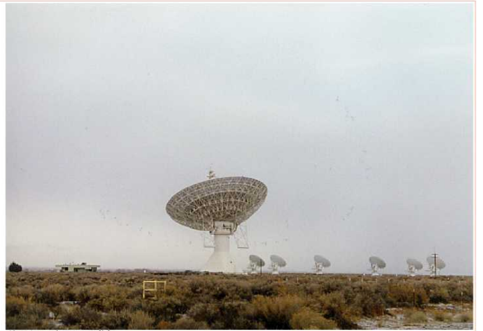
40-meter microwave dish.
