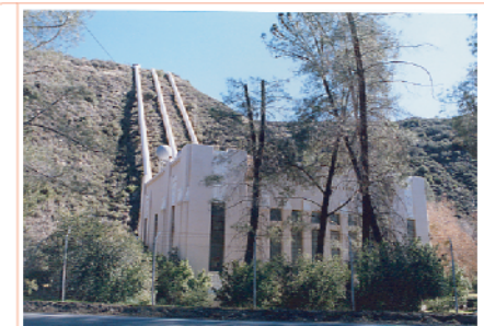
Power Station #2, San Francisquito Canyon.
