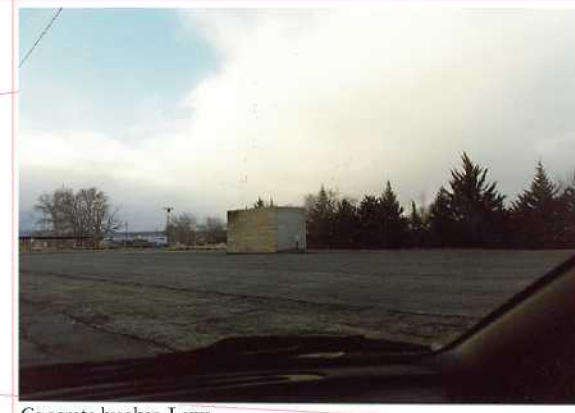
Concrete bunker, Laws.
