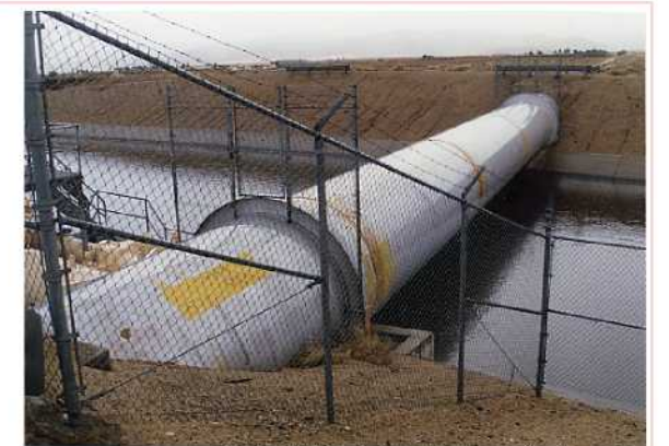
LA & California Aqueducts crossing, Neenach.
