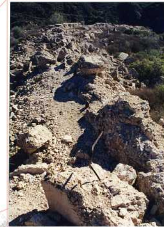
Pulverized concrete remains of the St. Francis Dam, San Francisquito Canyon.
