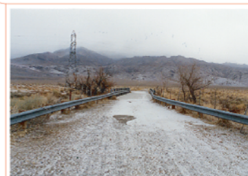
Ranch road at Owens River north of intake.
