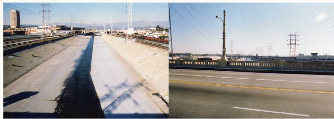
LA River from 1st Street, downtown. During dry times, the river doesn't even fill the central subchannel, seen below.
