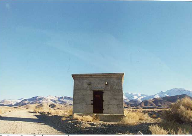
Bunker at Cerro Gordo access road.
