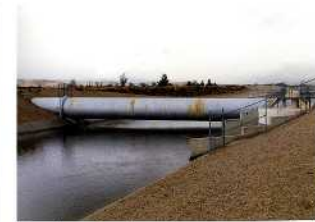
Los Angeles Aqueduct crossing the State Water Project channel in Neenach.
