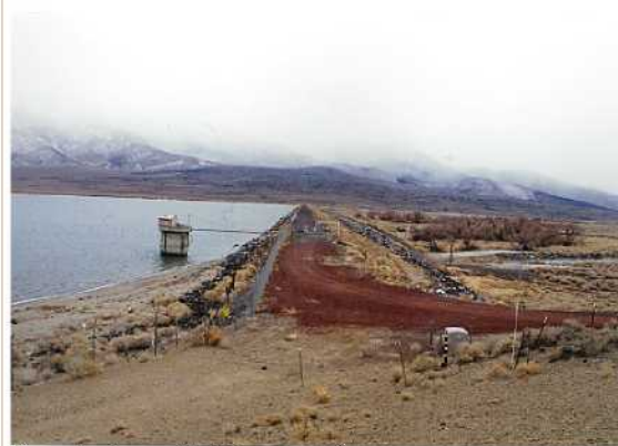
Tinemaha dam and holding reservoir.
