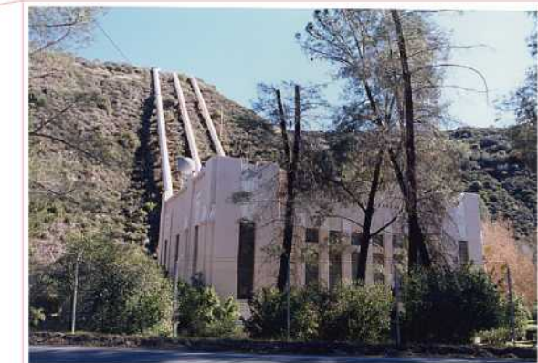
Power station #2 in San Francisquito Canyon.
