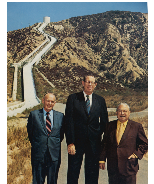
Cascades for Second Aqueduct, 1971 (Department of Water and Power).
